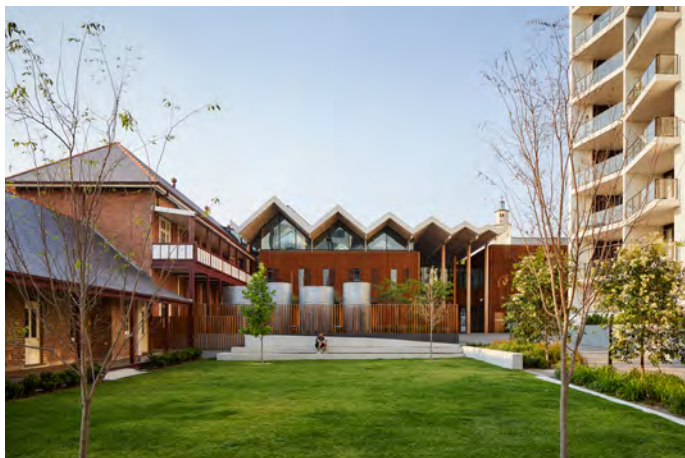
Figure 14. Water tanks in the children garden which harvest rain water for the gardens. (Image: Brett Boardman Photography)
