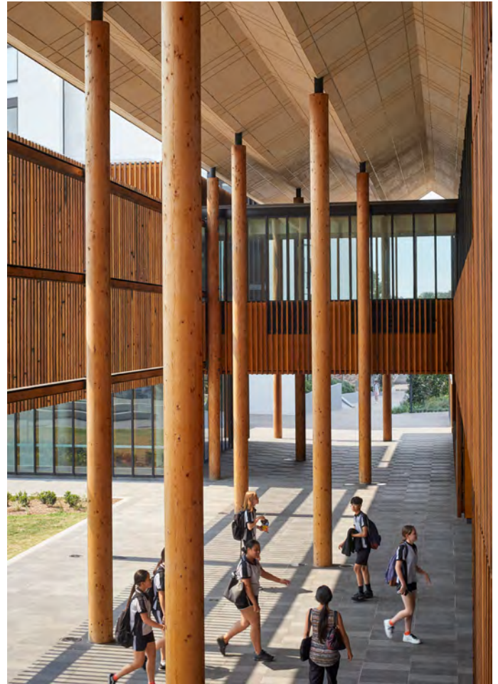
Figure 16. Solar shading of Hospital Lane and main entry by cantilevered roof and western timber solar shade. (Image: Tom Roe)
