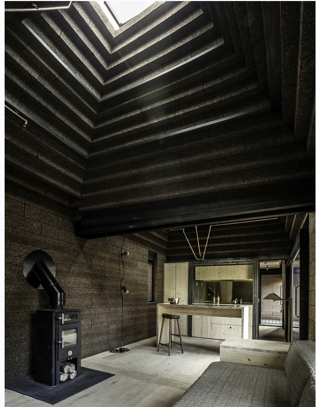
Figure 15. Cork House, London, by Matthew Barnett Howland with Dido Milne and Oliver Wilton. Built from stacked cork blocks with interlocking joints means the cork forms the structure, insulation and internal and external surface finishes. The house is estimated to have a whole life cycle carbon of just 15% of a typical new build (Crook 2019). (Image: Magnus Dennis)
