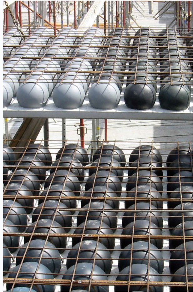
Figure 10. 'BubbleDeck' slabs can reduce the amount of concrete used. In the Mills Park community centre in Beckenham, Perth, the use of BubbleDeck reduced the need for 250m 3 of concrete as compared to conventional slabs (BubbleDeck 2018). (Image: BubbleDeck)
