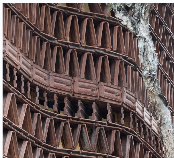
Figure 13. The Beehive, Sydney, by Luigi Rosselli Architects and Raffaello Rosselli Studio. At this office building in Surry Hills, waste terracotta roof tiles were stacked in a variety of patterns to create solar shading for the western facade. The same tiles were also used internally to create bookshelves. (Image: Ben Hosking)
