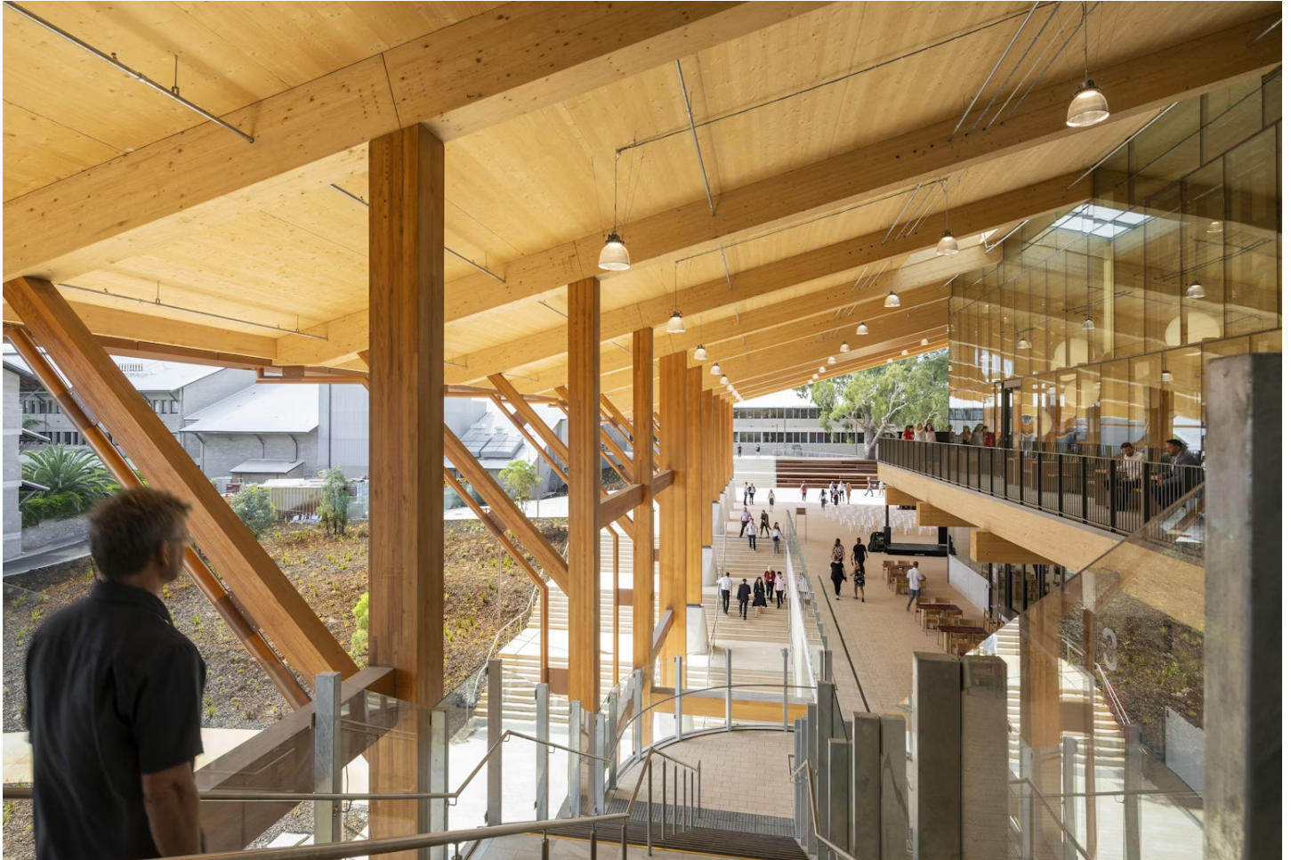
Figure 14. Boola Katitjin by Lyons with Silver Thomas Hanley, Aspect Studios, Officer Woods, and The Fulcrum Agency. Big open circulation spaces open to the environment allowing for an energy efficient mixed mode ventilation strategy. Hardwood GLT columns support softwood GLT beams and a CLT roof. Columns and beams are diagonally braced to ensure both free standing columns and support of substantial roof overhang. K-Braces delivered the majority of the lateral stability system and wide roof overhangs provide shading and protection of external timber elements. The hardwood columns sit on concrete plinths. This is good durability practice to elevate timber off the ground. (Image: John Gollings)
