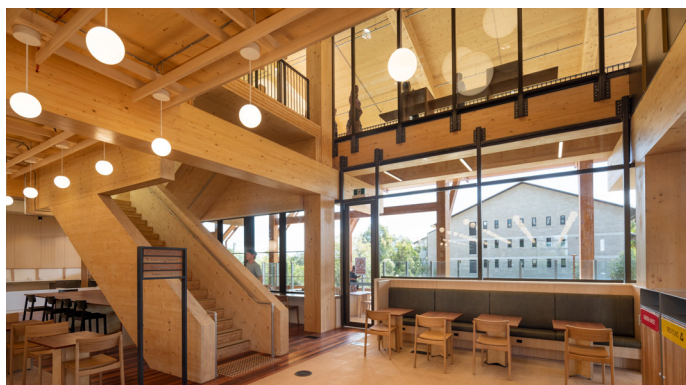
Figure 15. Boola Katitjin by Lyons with Silver Thomas Hanley, Aspect Studios, Officer Woods, and The Fulcrum Agency. Exposed timber elements require a well-considered services reticulation strategy. Services are often surface mounted and penetration through structural elements should be coordinated during the design phase and integrated into manufacturing process prior to site assembly. For Boola Katitjin, the services reticulation was provided through an Under Floor Air Distribution system (UFAD) which required a 600mm access floor across the project. This allowed maximising the beautiful visual exposure of the CLT soffit. (Image: John Gollings)
