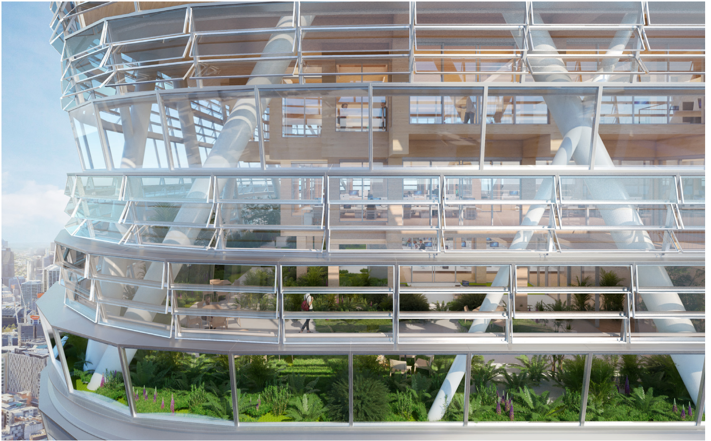
Figures 5 and 6. Atlassian Central, Sydney NSW by BVN SHoP Architects. Co-owned by Atlassian and Dexu. Sectional renders of the Atlassian Central building showing the mass timber-framed 'neighbourhoods' sitting in between the main steel structure. (Images courtesy of BVN SHoP Architects/Dexu)
