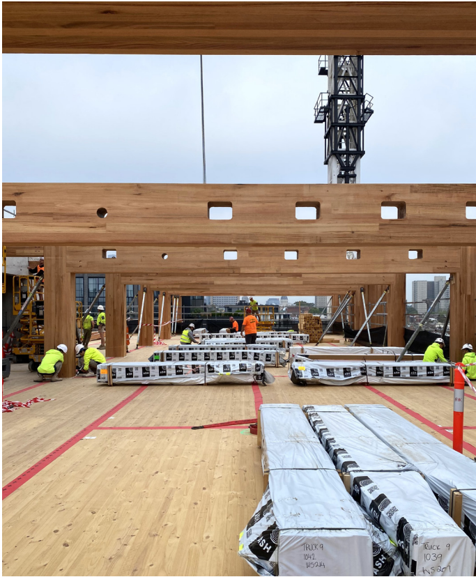
Figure 11. MASSLAM hardwood columns and beams positioned on live deck and lifted into position. Services penetration was coordinated up front and cut in factory prior to installation. (Image: Australian Sustainable Hardwoods)
