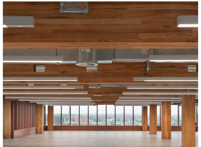
Figure 13. Completed floor which internally exposed hardwood GLT columns and beams. (Image: John Gollings)T3's timber approach represented a 34% reduction in estimated upfront carbon emissions versus the same building when designed with a conventional concrete frame as calculated by the engineers, Aecom, using the Green Star upfront carbon emission calculation guide 2022. The estimated carbon reduction calculation is based on class A1- A5 EN15978, from raw material to construction on site.
