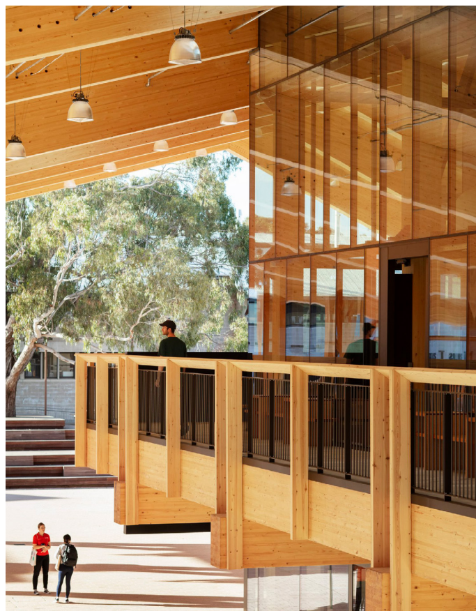
Figure 16. Boola Katitjin by Lyons with Silver Thomas Hanley, Aspect Studios, Officer Woods, and The Fulcrum Agency. Internal balconies and walkways suspended off cantilevering GLT beams. Balustrades and handrails supported from the beam edge with a very simple bolt on connection. The combination of different materials with timber elements requires a good understanding of the materials’ behaviours and the required tolerances in the interfaces, ie timber to glass or timber to steel. Materials expand and shrink differently under different conditions. (Image: John Gollings)
