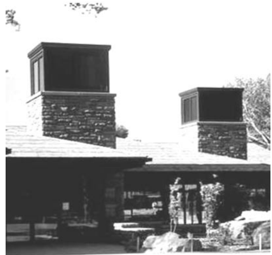
Figure 11. Evaporative Cooling Towers, Zion National Park, Utah, USA (courtesy of D Balcomb).
