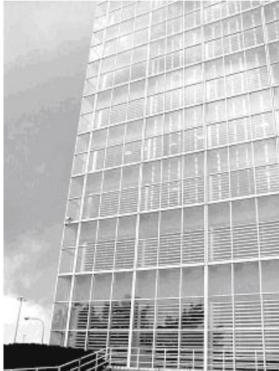
Figure 18. Occidental Chemical building utilising a double envelope and convective loop (photo: M Luther)
