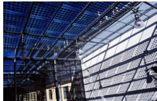
Figure 7. Glass encapsulated photovoltaics in library roof
