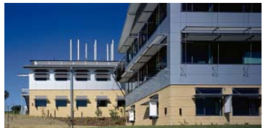
Figure 3. Elevation detail showing shading devices on offices and laboratories
