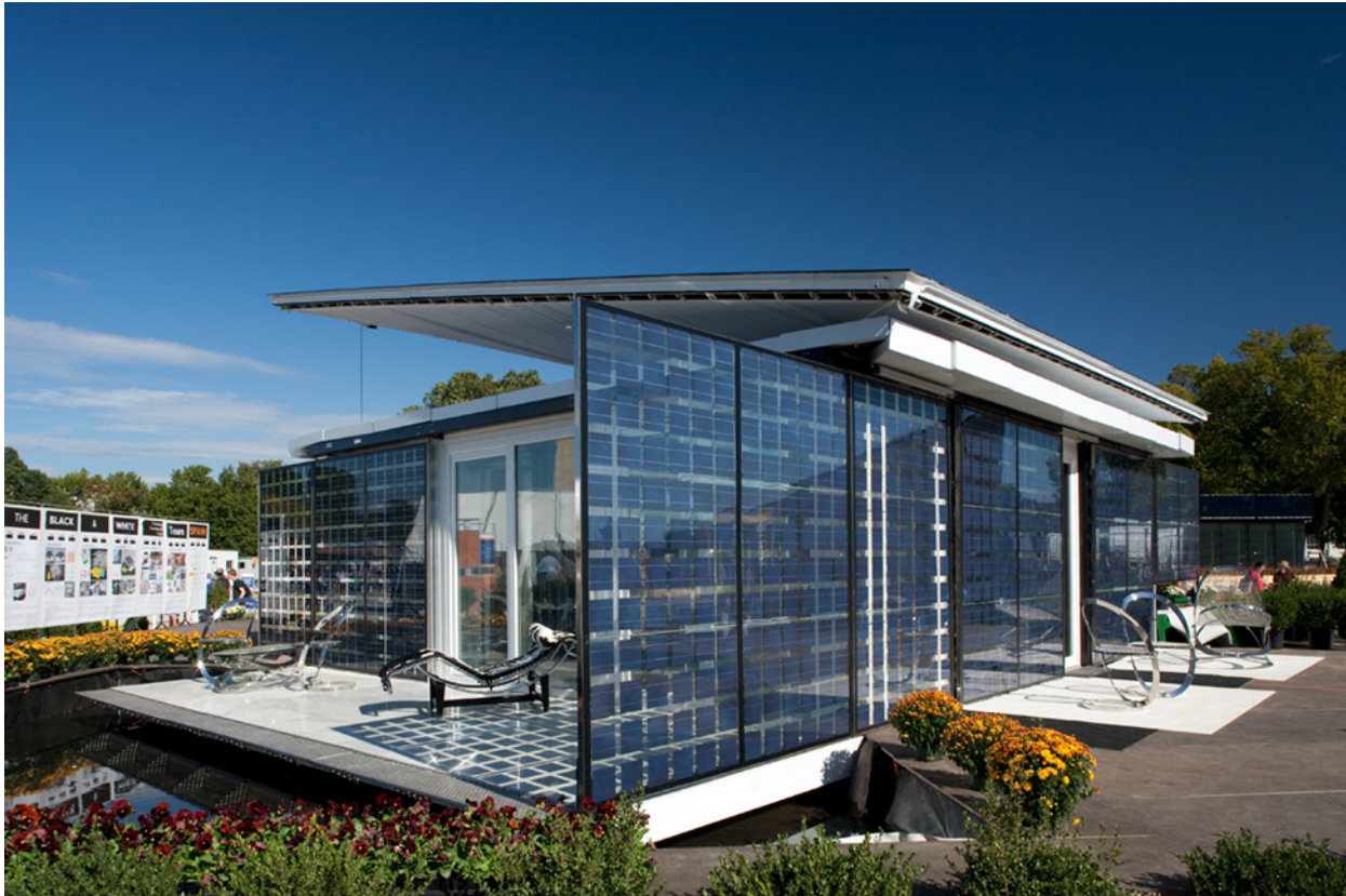
Figure 3 Surfaces incorporating PV cells can provide shade while generating electricity.
