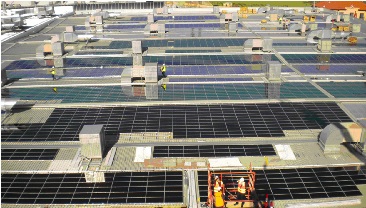
Figure 8 1 MW roof-mounted PV system at Adelaide Showgrounds, using cadmium telluride solar cells (Image: First Solar)
