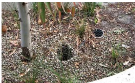
Figure 20. Short-circuit from tree stake Hole in filter media after tree stake removed visible in centre of photograph (Source: EDAW)
