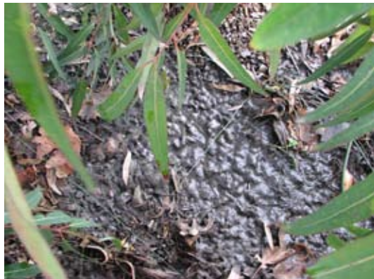
Figure 17. Sediment build-up on top of and within gravel mulch (Source: EDAW)
