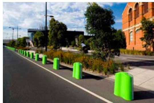
Figure 16. Batmans Hill Drive bioretention swale with traffic bollards
