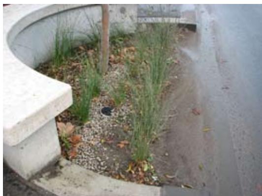
Ag pipes visible at garden surface
