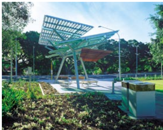
Figure 8. Bus shelter with PV cells
